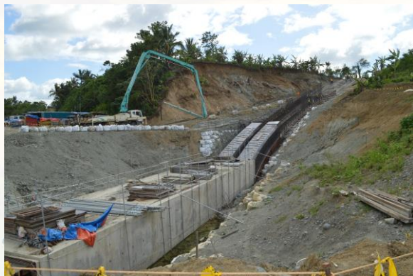
Siphon #2 Brgy. Toyungan, Calinog, Iloilo
